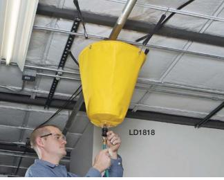
Installation is easy – simply hang from overhead pipes.
