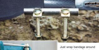
pipe and tighten the clamp.
